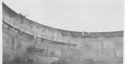
WORKMEN SEEM dwarfed by the tremendous circular sweep of the tank's inner wall. The plates that make up the sides have smaller thicknesses as they approach the top.
